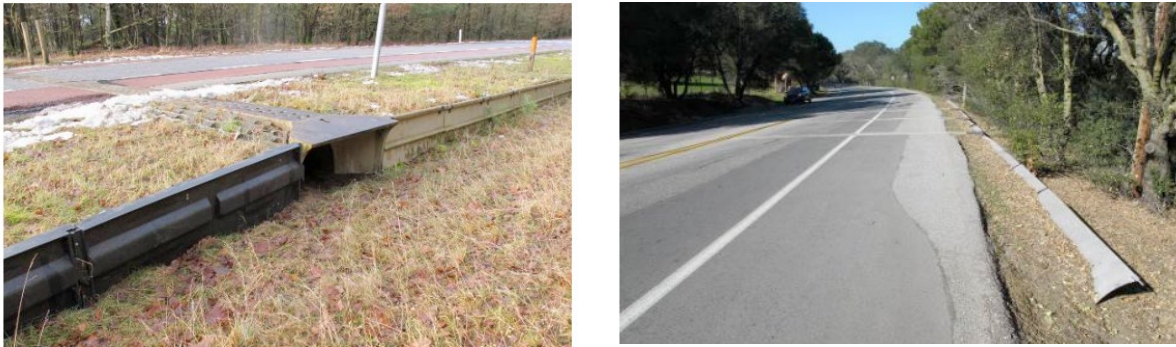
Figure 13. Two examples of directional barriers; Left: showing built-in overhang; Right: showing angled to ground (Langton and Clevenger 2021)
