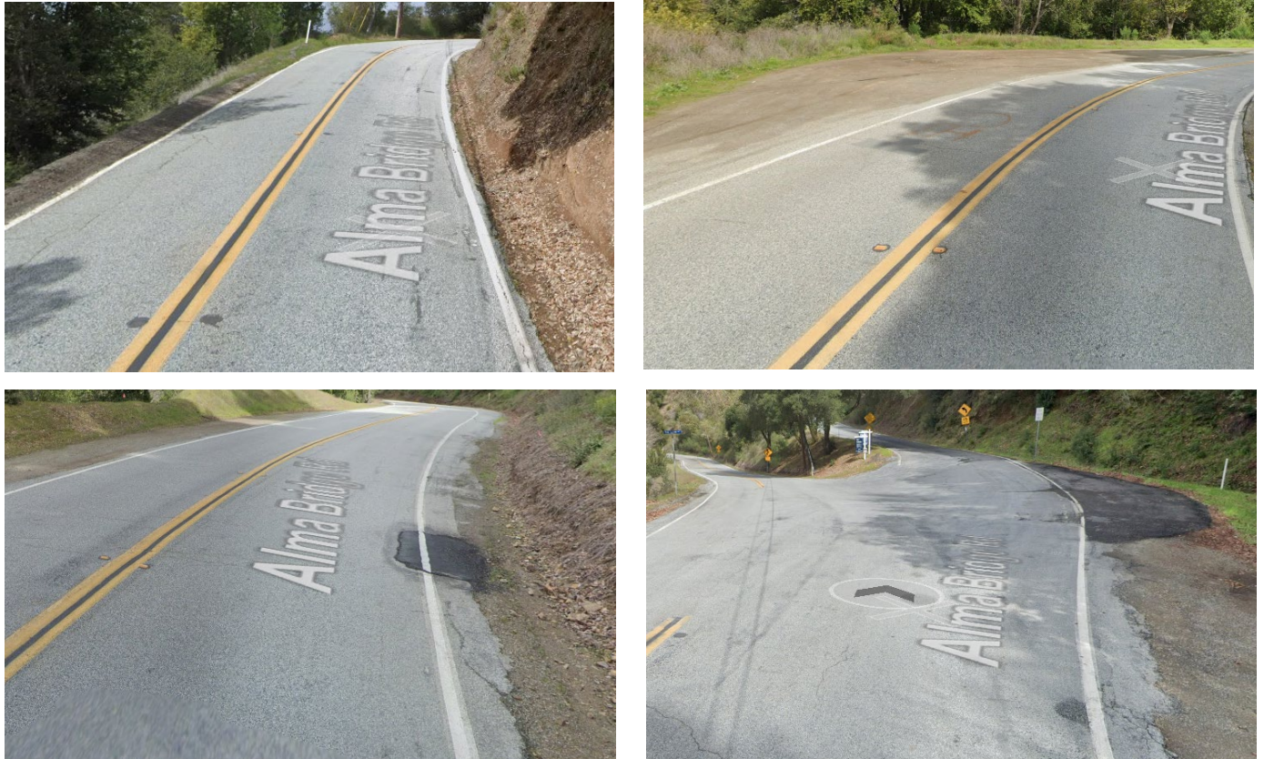
Figure 14. Examples of road shoulders and unofficial turnouts on Alma Bridge Road. Top Left: Example of 0-1 foot shoulder; Bottom Left: Example of 1-2 foot shoulder; Right Top and Bottom: Examples of unofficial turnouts (Source: Google Maps)
